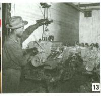
frequently damaged in shipping, and was later reallocated for installation at the car assembly plants. Note the "log" exhaust manifolds, no oil filter pad, and no side motor mount bosses. Copyright 2005 GM Corp. Used with permission, GM Media Archive
